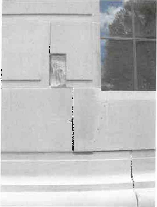
Other repairs included various spall repairs, pinning and epoxy injection of larger cracks and lifting and pinning keystones over windows.
